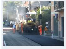
The asphalt used is made of a relevant percentage of recycled rubber with high sound absorption performances (3-4 dB less than conventional asphalt in European applications in urban areas at 40-45 kmh speed)
