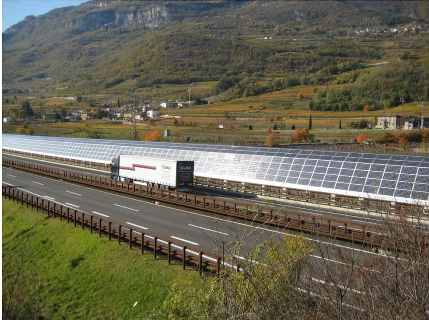
Figure 14: Noise barrier equipped with photovoltaic modules installed on the Italian Motorway A22 “del Brennero” [14]
