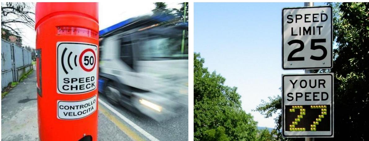
Figure 16: different types of speed reduction devices: speed checker (on the left) and radar speed sign (on the right)
